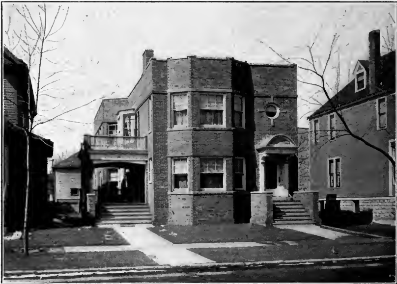
RESIDENCE IN OAK PARK.
